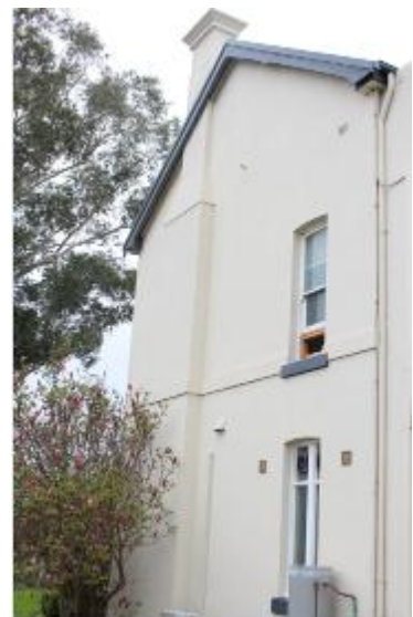
Figure 17: East facade of subject building.
