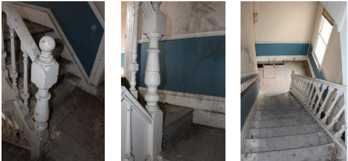
Figure 25: Space F.1 - Stair Hall
