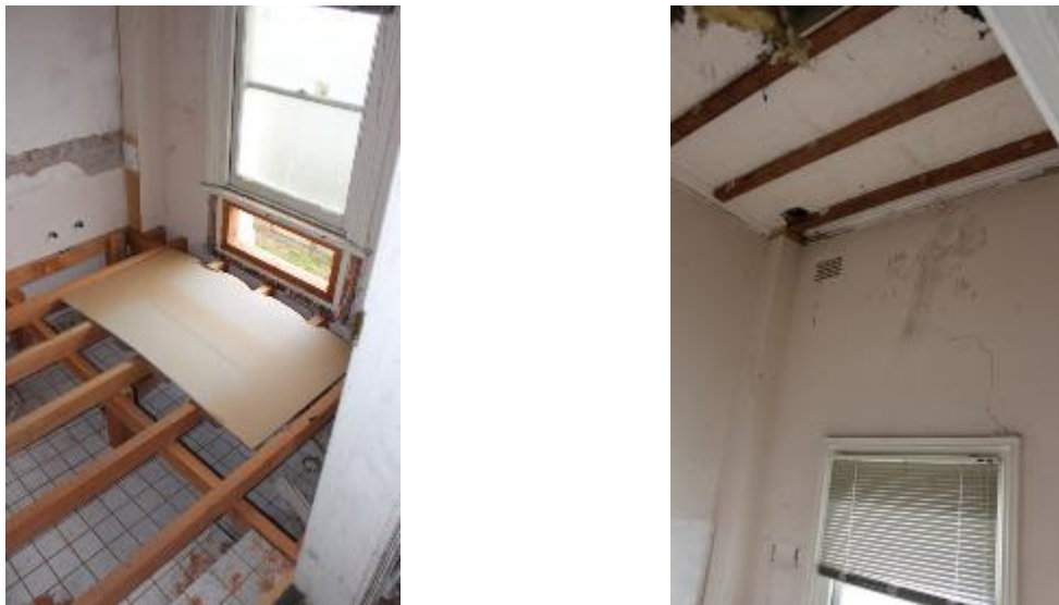
Figure 32: Space F.6 - Bathroom
