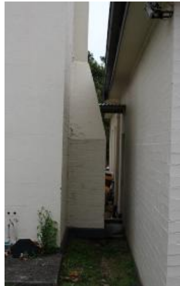
Figure 15: Junction with subject building and rear annex viewed from east
