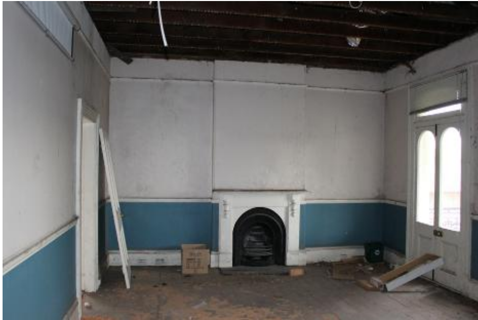
Figure 29: Space F.2 - Bedroom 1 & French Doors to Verandah
