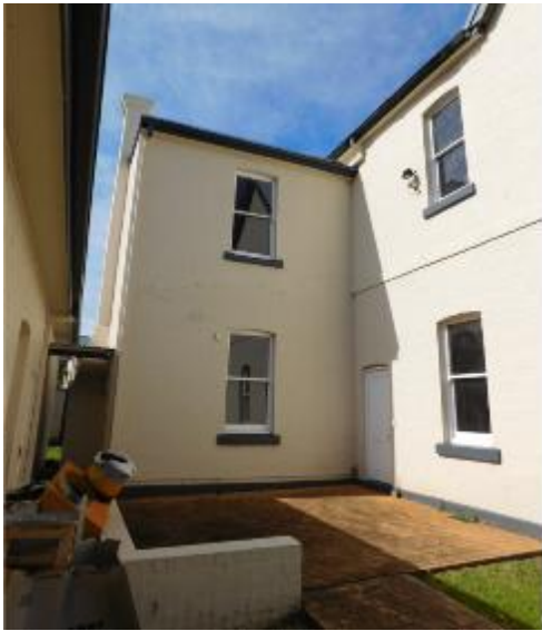
Figure 14: Subject building with rear kitchen wing, viewed from west
