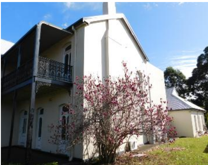
Figure 16: East facade of subject building viewed from entry garden, looking north
