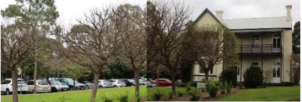
Figure 11a: Subject building - Entry facade (south) & pathway to front door
