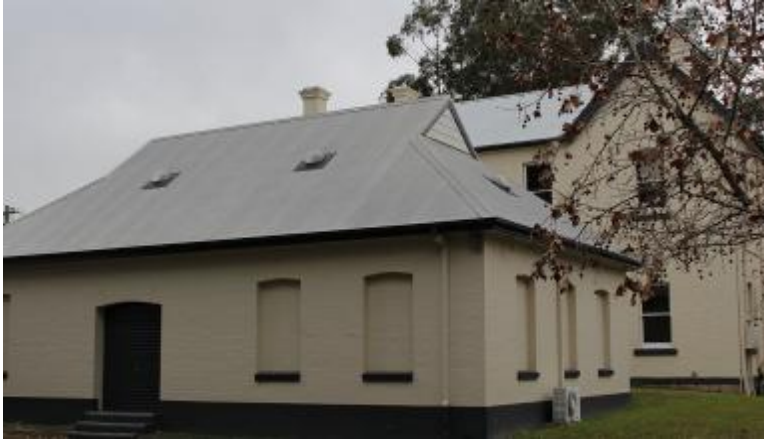
Figure 18a: Rear north facade and recent annex.
