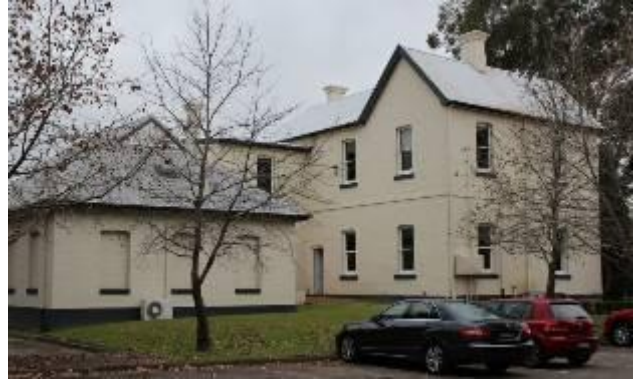
Figure 13: Subject building – North corner, including recent annex viewed from property car park
